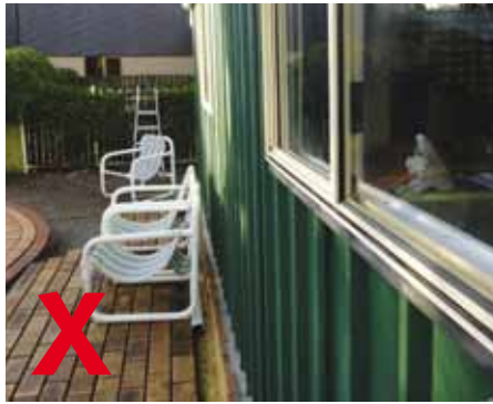
Windows that provide easy access to the pool area must be secured.
