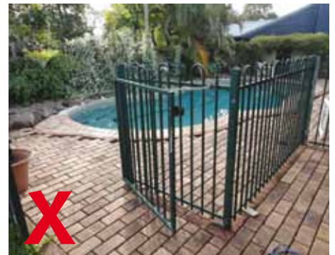
A gate cannot be tied or propped open and must self-close from any position.
